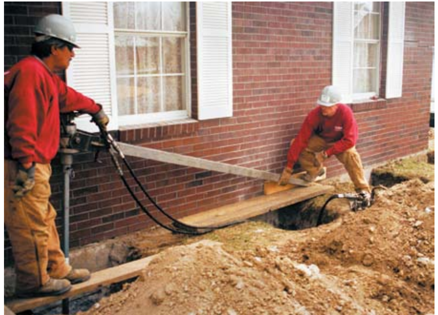
Helical pile installation by hydraulic driver
