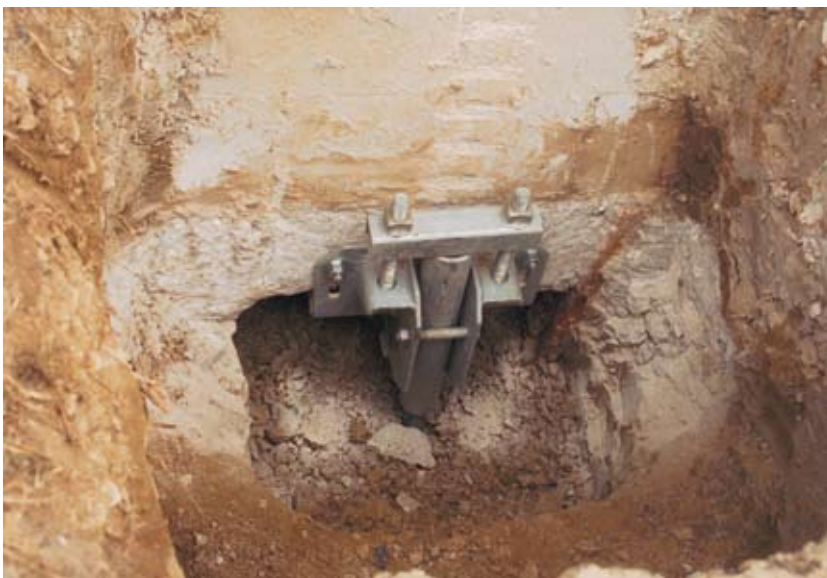
Completed helical pile and bracket
