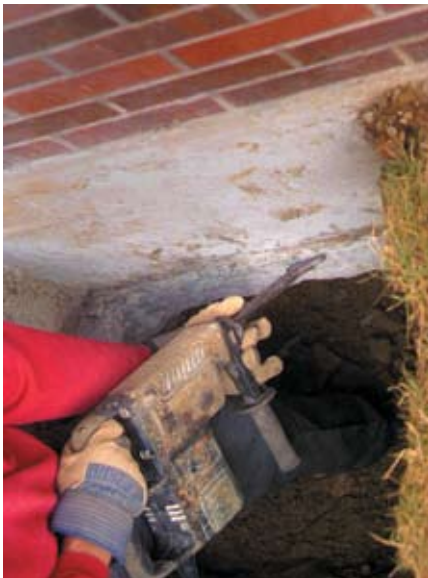
Chipping notch out of foundation footing for bracket attachment
